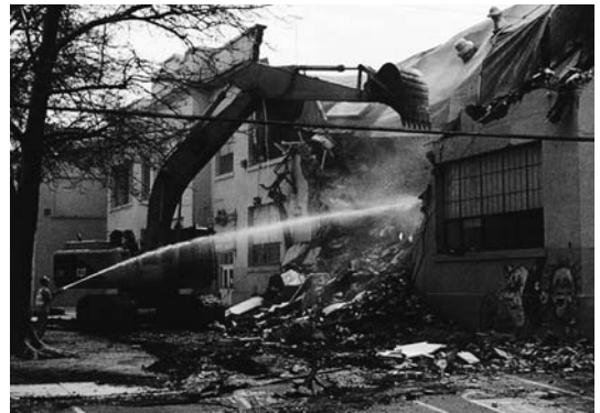
demolition in progress
